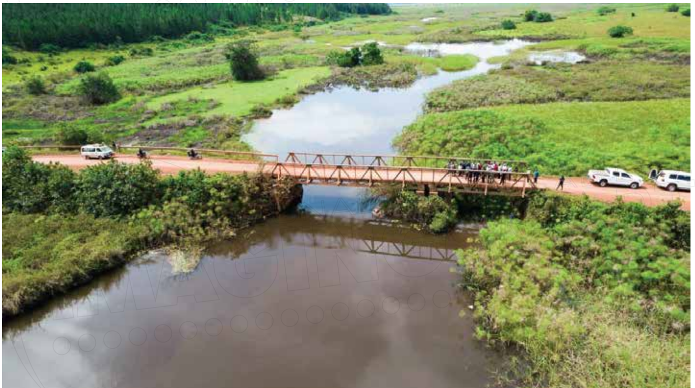
Underestimating project costs can arise from failure to visit and assess thoroughly challenges of remote sites: Government officials visit an old bridge set to be replaced by a new one over River Ngono at Kyanyabasa, Bukoba Rural District. [Photo: Tanroads]
